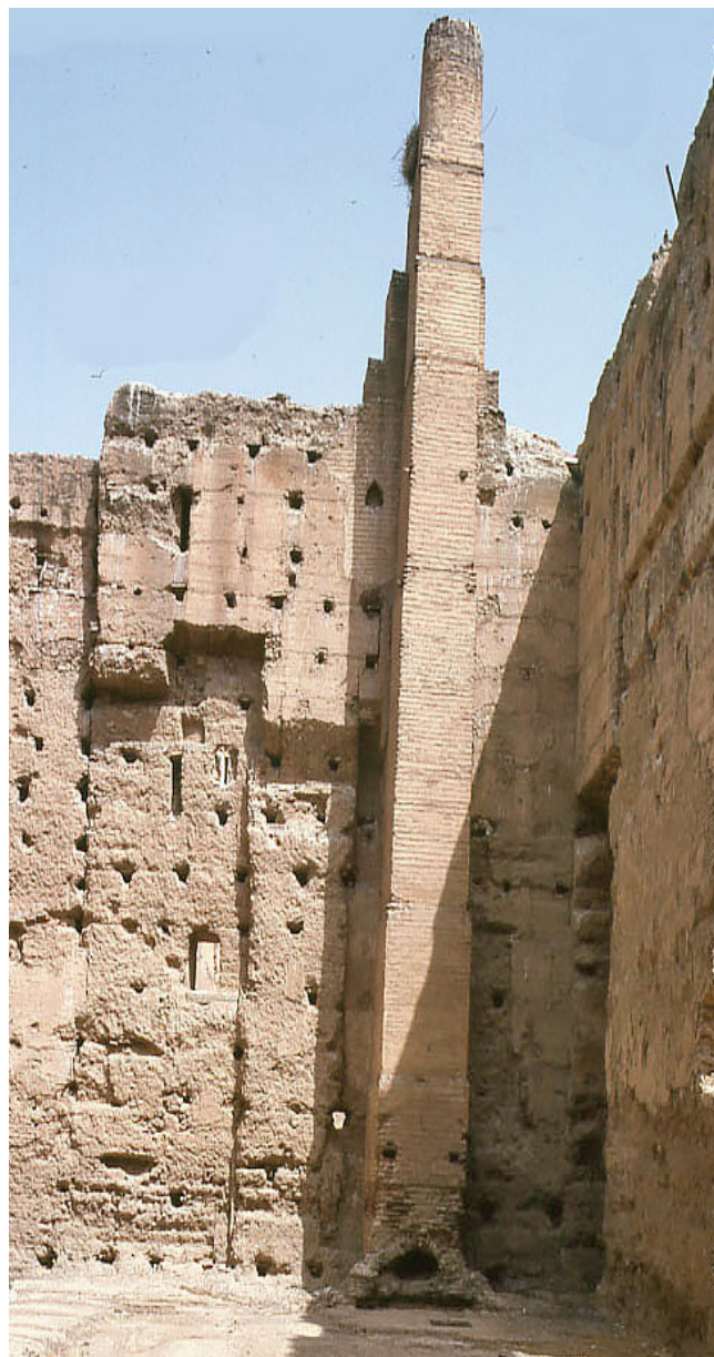
Figure 4: Tall chimney leading from the furnace shown in Figure 3. This would have created a great updraft, requiring careful control of the air entering the furnace as Al-Djazznā'i instructed. It would also have been necessary to remove the noxious fumes from the refining operations.
