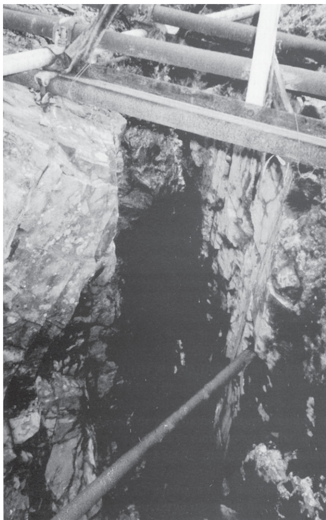
Figure 1: The forebreast of this stope in a Bronze Age mine at Copa Hill, Cwmystwyth, reveals a solid rib of galena from top to bottom, with every indication that it was the mineral worked. Note the smooth slickensided wall of the lode. (Excavation by the Early Mines Research Group)
