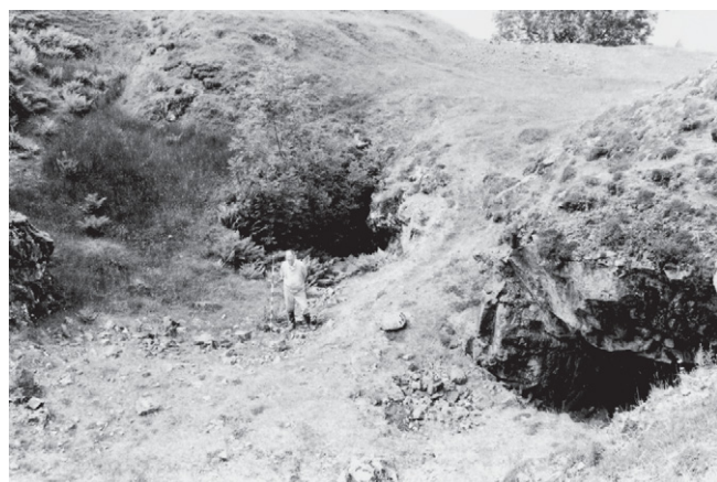
Figure 5: Looking across the open working to the north-west. The vertical shaft in the middle distance originally connected the openworking with the entrance adit (see Fig 3).
