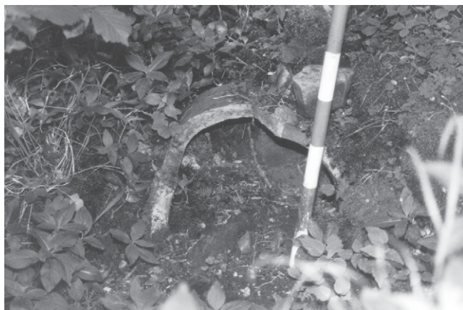
Figure 14: Earthenware pipe at junction of flue from second terrace with main acid flue.
