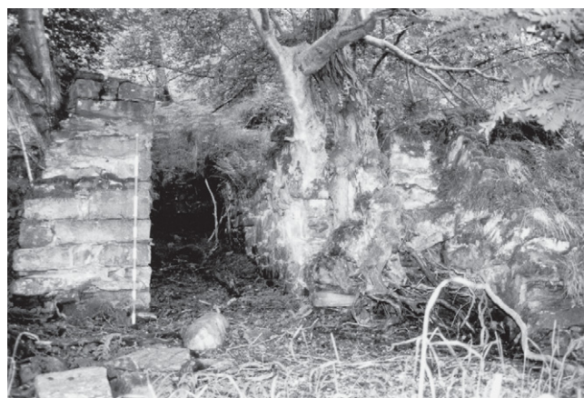
Figure 9: View of the furnace looking SE. The buttress on the right side of the photograph is believed to have carried rails as part of the charging system.
