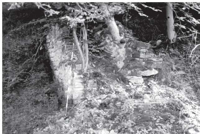
Figure 13: The main acid flue.
