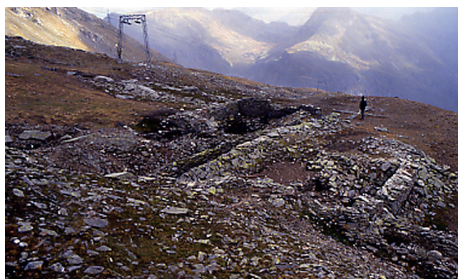
16th-17th century gold mines on Kreuzkogel, Sportgastein. Note the roof slabs of the Schneekragen covered way linking the mine buildings on the right with the adit entrance to the left (photo P T Craddock 1987).
