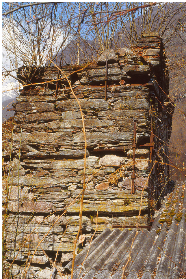
Figure 9: The Norwegian blast furnace at Fiumenero was rebuilt in the 19th century in the Bergamasque furnace style, although its crucible was circular rather than square.
