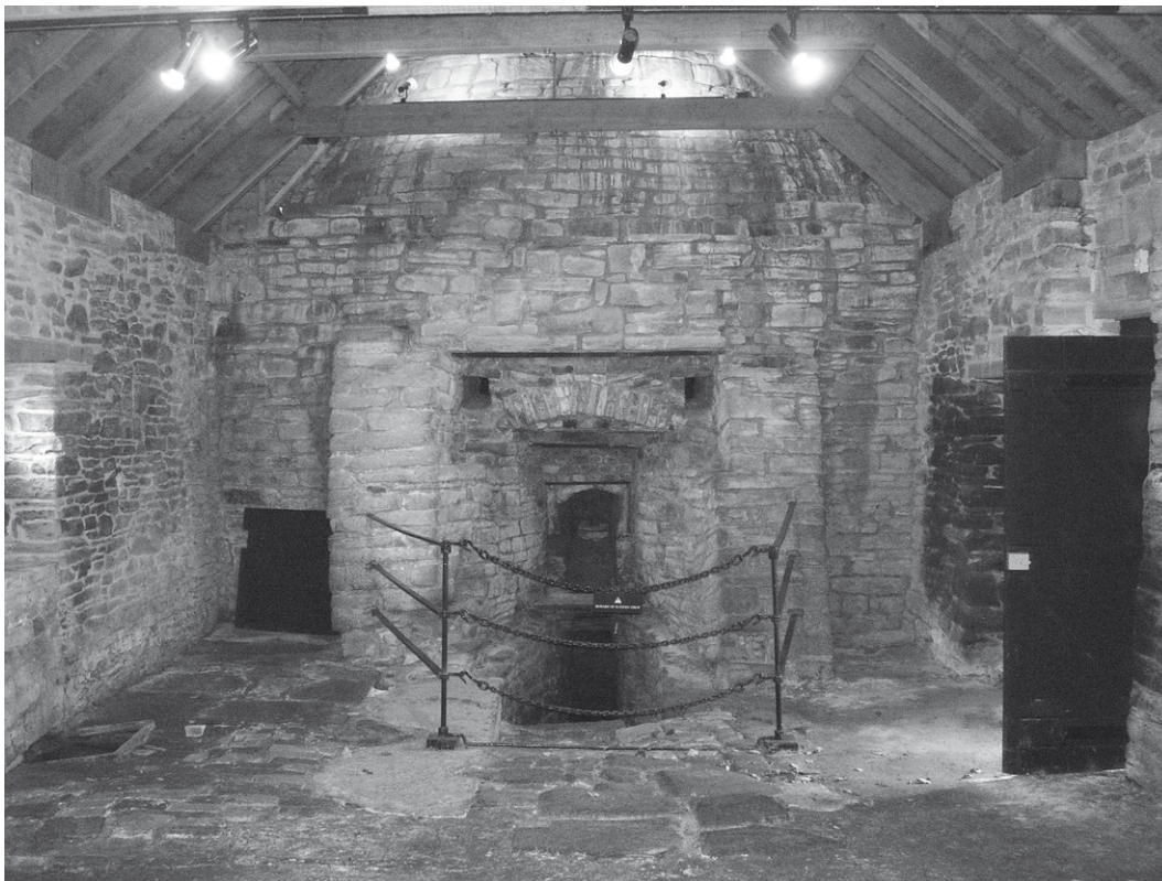
Figure 9: Derwentcote: south face of furnace within ancillary building. In use, the ashpit (behind modern railings) would be covered iron plates, and without the modern lighting the red glow would form a strong visual focus between the projecting buttresses (photo Paul Belford).
