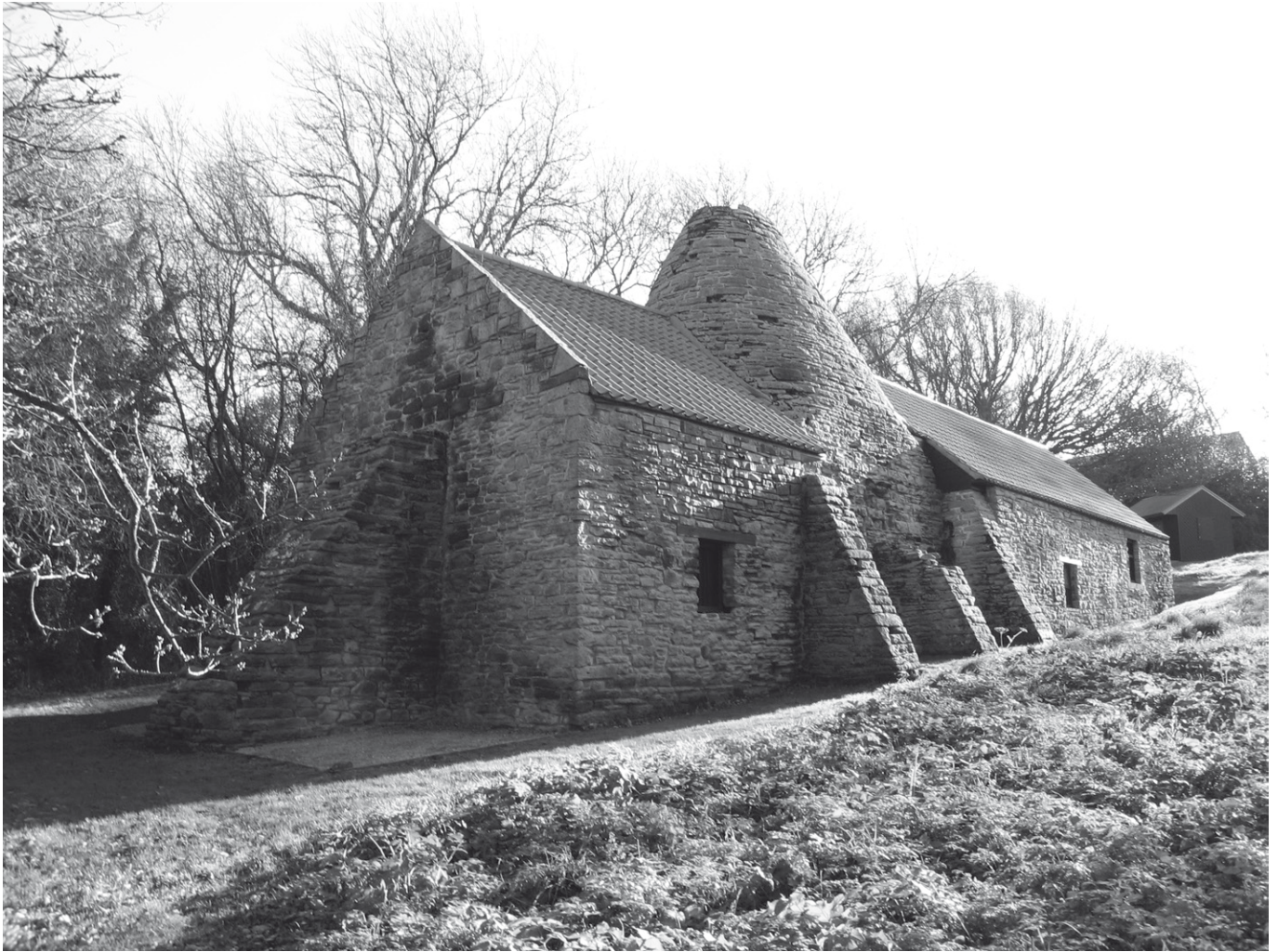
Figure 1: Derwentcote furnace in 2007; the ‘reverse-crowstepped’ north gable (left) forms the only overtly non-functional element. The pantile roof is a modern replacement—the original handmade pantiles would have created a less coldly-uniform appearance than their modern machine-made replacements.
